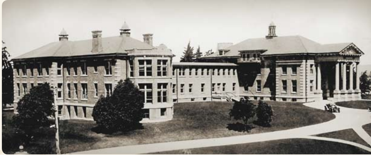
Samuel Merritt Hospital, 1909.
